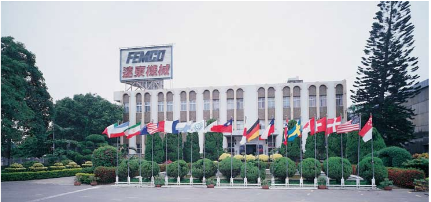
Headquarters at the How-Hu Factory plant in Chiayi, Taiwan.
